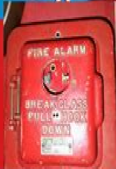
Vintage 1965 Simplex Type-4246-2 Fire Alarm Control
