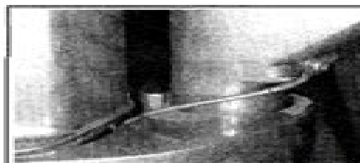
Fig. 28 One of the many lead wires used to connect bracketed parts. Lead wires are used as an assist in reducing corrosion
